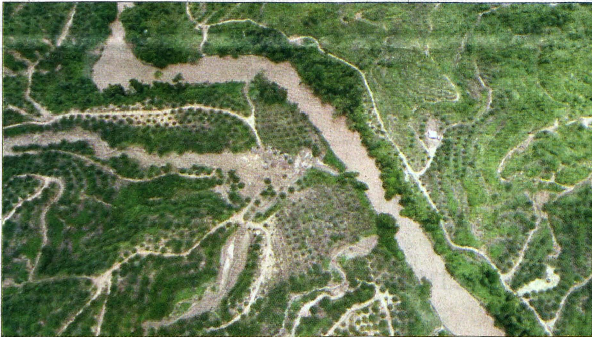
Signs of the mudslide making its way to the workers’ quarters beside the Sungai Pinangah. Picture courtesy of Peter Chau for UMS Natural Disaster Research Centre.
