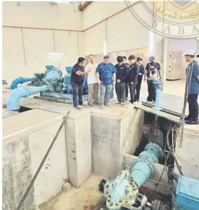
In May, Shahelmei conducted a working visit to the UMS pump house near the R13 tank.
